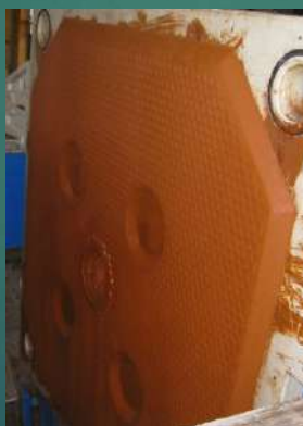
压滤泥饼 Filter mud cake
