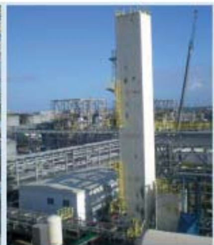
Nickel Refinery Plant Site
