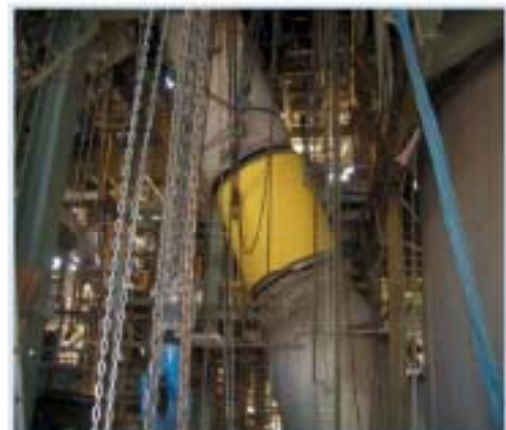
Catalyst Standpipe on Installation
