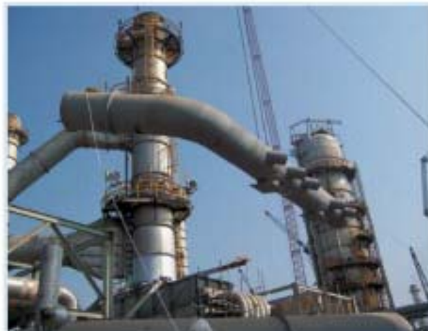
VTL under Installation
