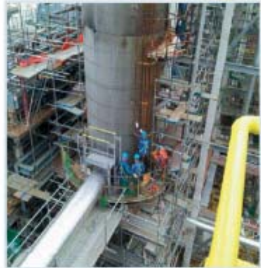
MHC Revamping Site
