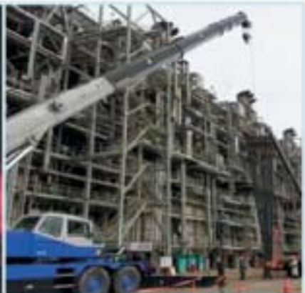
Lifting of New Coil Bundle
