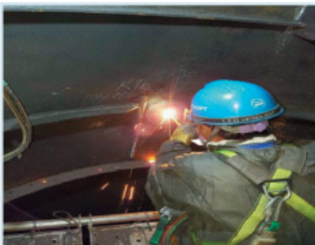
Nozzle on Modification
