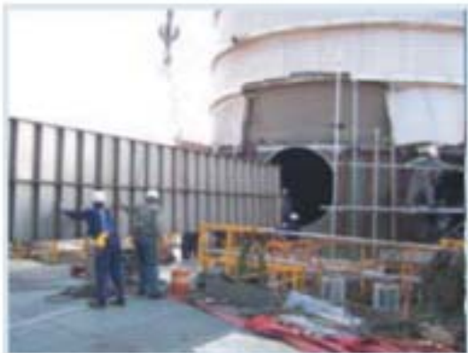
Installation of Schopentoeter
