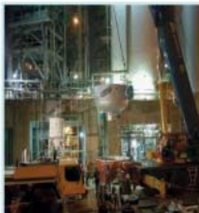
Install. of New Cooler B/H
