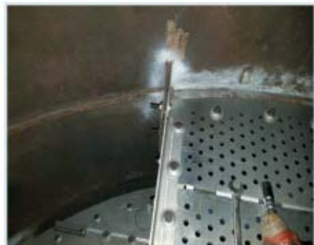
Tray under Installation
