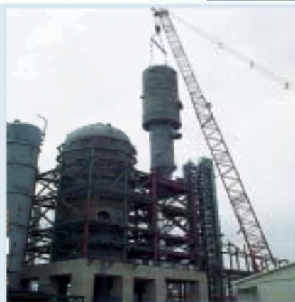
Installation of Reactor
