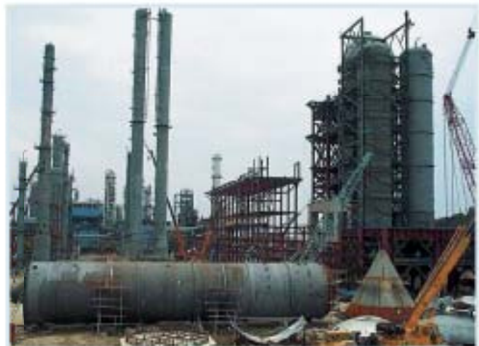
CPC RFCC Installation Site
