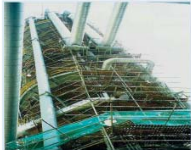
No.2 Crude Column on Revamping Work
