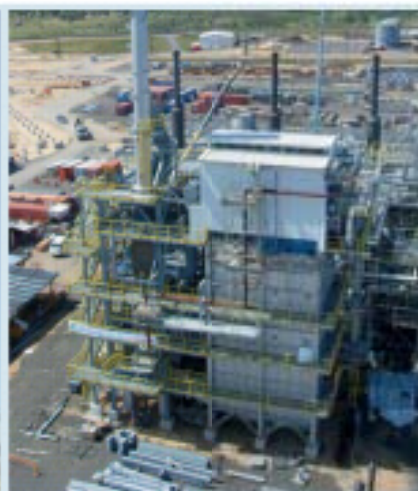
Installation of Reformer
