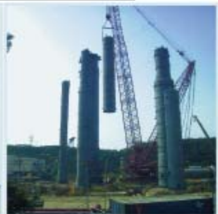
Fractionator on Installation
