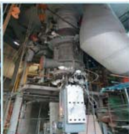
New Plug Valve Replaced
