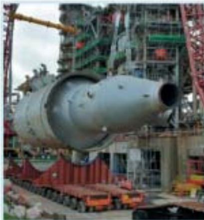
Loading of Old Reactor
