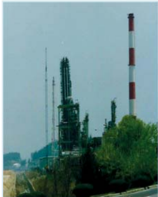
Overall View of S-Oil No.2 Crude Column
