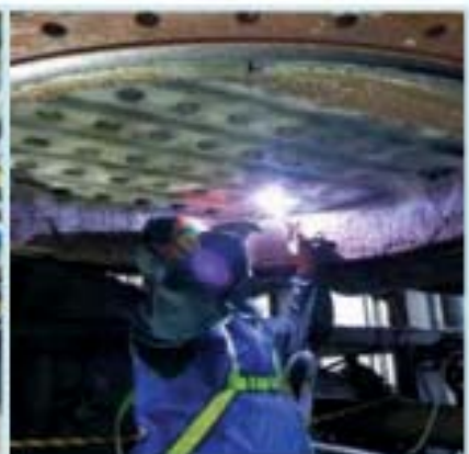
Bottom TLE on Repair Work
