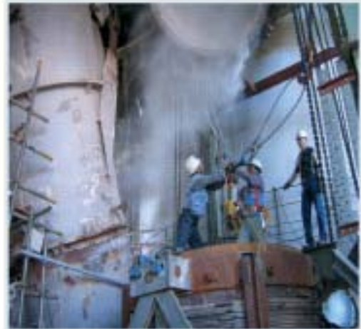
Existing Expansion Joint Line under Disassembling
