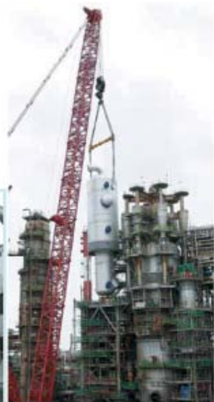
New Reactor on Installation
