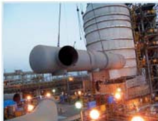
Installation of Schopentoeter
