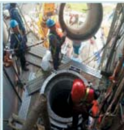
Install. of New Spent Line
