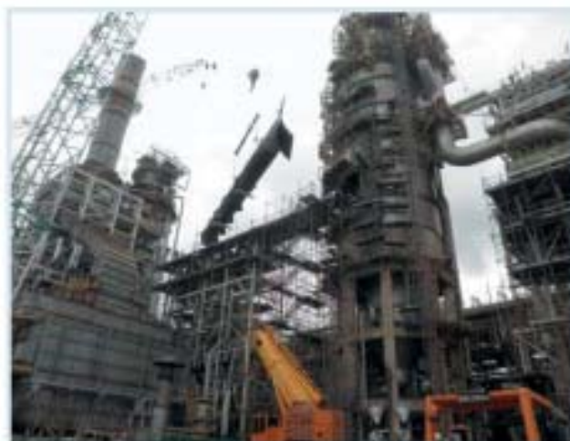
Preparation for Installing New VTL
