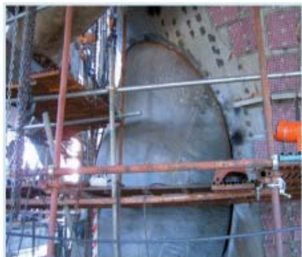
Transfer Nozzle under Installation
