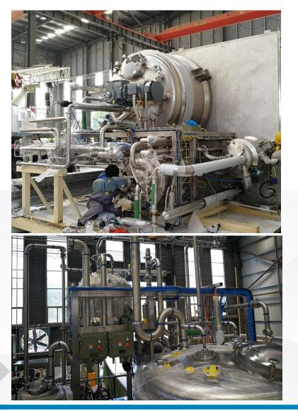
Main mixer skid is composed of 5m3 main mixer vessel, 1m3 quat premixer vessel, 2m3 fabclean premixer, lobe pumps, heat exchanger, MCC Panel, valves, piping.
