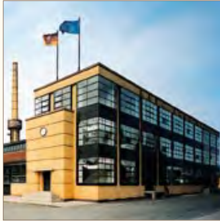
Fagus Factory, constructed by Walter Gropius in 1911
