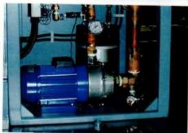
Drain the water from the manual valve located in front of the pump
