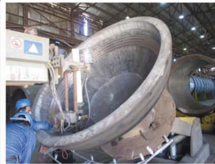
Weld Overlay : Head (Head Cladding Column & Boom - Positioner) Weld Overlay
