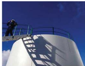
South Azadegan Oil field Water Storage Tank - 2016
