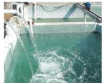
Crystal Clear Condensate from Distillery Industry ZLD Plant
