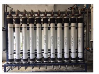
Dedicated backwash pumps connected to a backwash water source will be provided as part of the equipment. Modules will be filled with the filtrate before scouring with them air. A suitable acidic/alkaline cleaner dosing and chlorine dosing system will be provided to dose chemicals as required during air scouring of the Ultra-filtration membranes. The dosing sequence will be controlled by the PLC and will be done by means of metering pumps to ensure accurate and optimum dosing.
