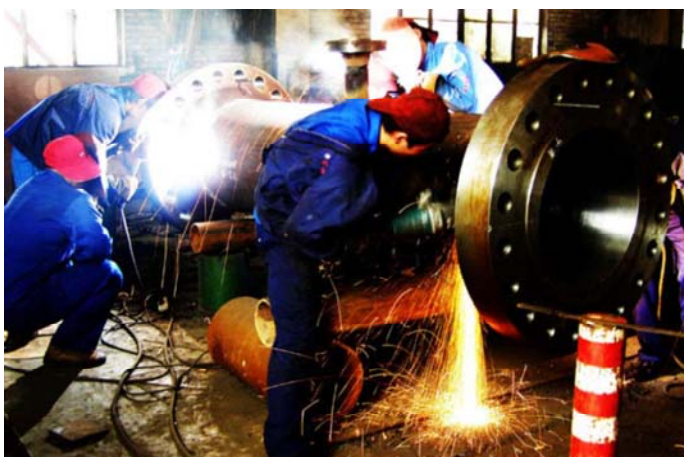
手动焊接 Manual welding
