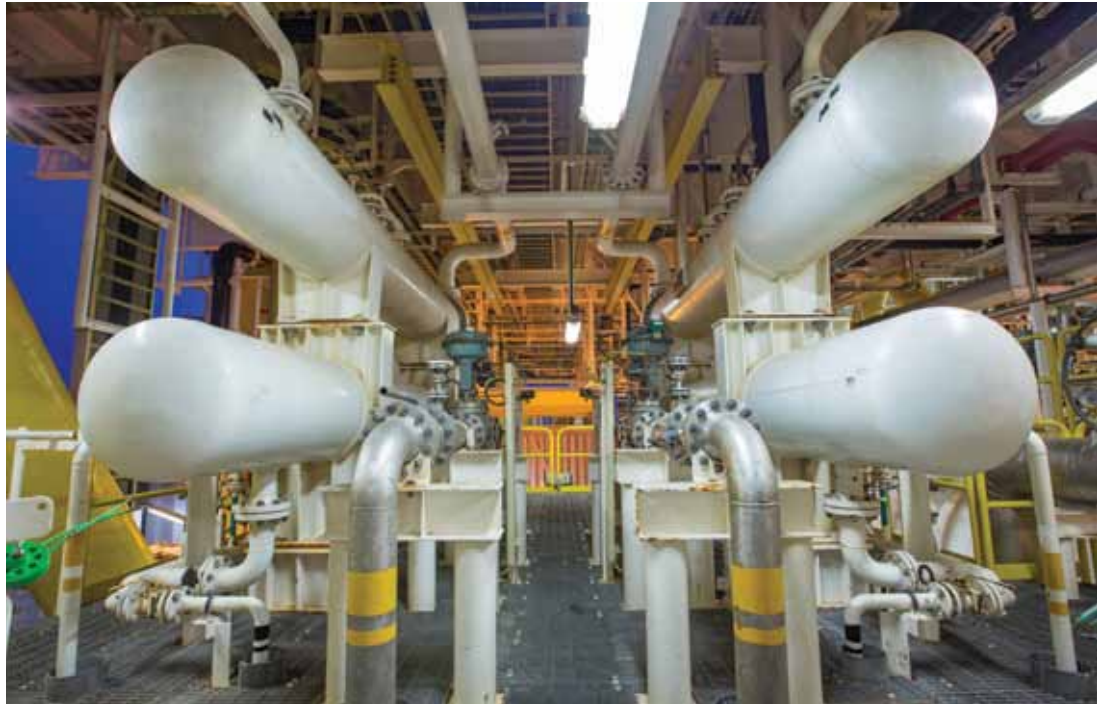
⚡ Heat exchanger shell and tube at offshore oil and gas central facility.
