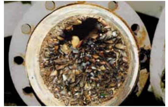
➤ The amine-based product penetrates biological membranes and the biofilm, disrupting the coherence of the biological structure and ultimately proving fatal for micro- and macro-organisms such as those shown in this heavily fouled water inlet.
