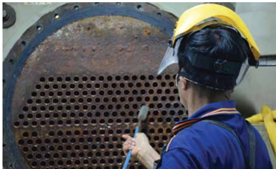
⚡ Mechanic is cleaning condenser tube of Chiller - HVAC System.
