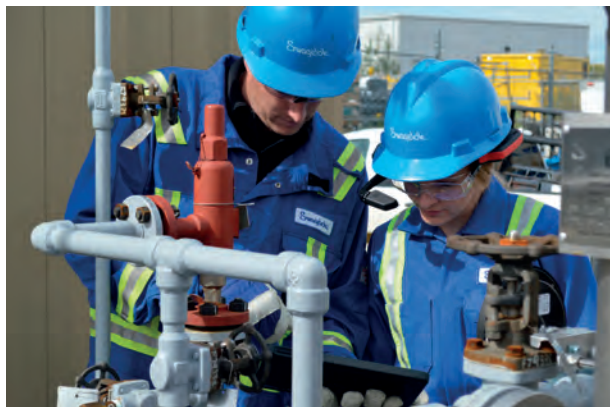
Figure 1. Chemical plants and refineries must continually validate process conditions and fluid compositions to ensure quality control throughout their facilities.
