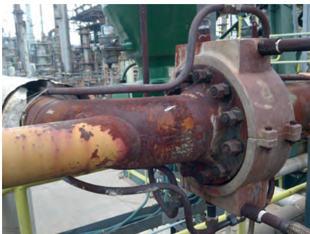
Figure 4. Bolt-on jacketing for flanges.
