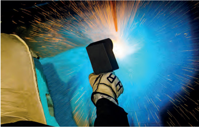
Figure 3. A technician applying HVTS cladding to a substrate.
