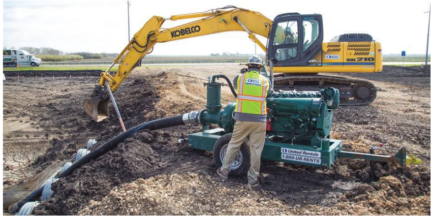
IMAGE 1: Most construction projects that involve excavation require the removal of groundwater or surface water. (Images courtesy of United Rentals)
