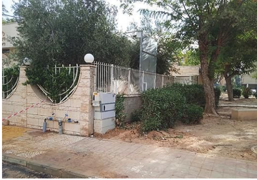
IMAGE 1: The main water supply pipe comes from under the ground (Images courtesy of the author)
