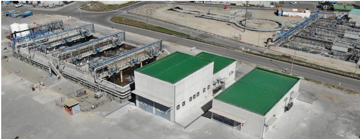
Figure 1: DEMON installation at a municipal wastewater treatment plant.
