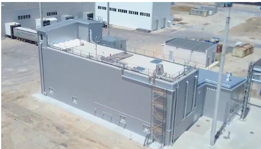
Figure 2: DEMON installation at a food processing facility.
