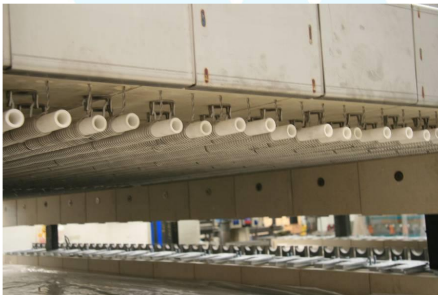
Top heating elements of last 2 heating modules
