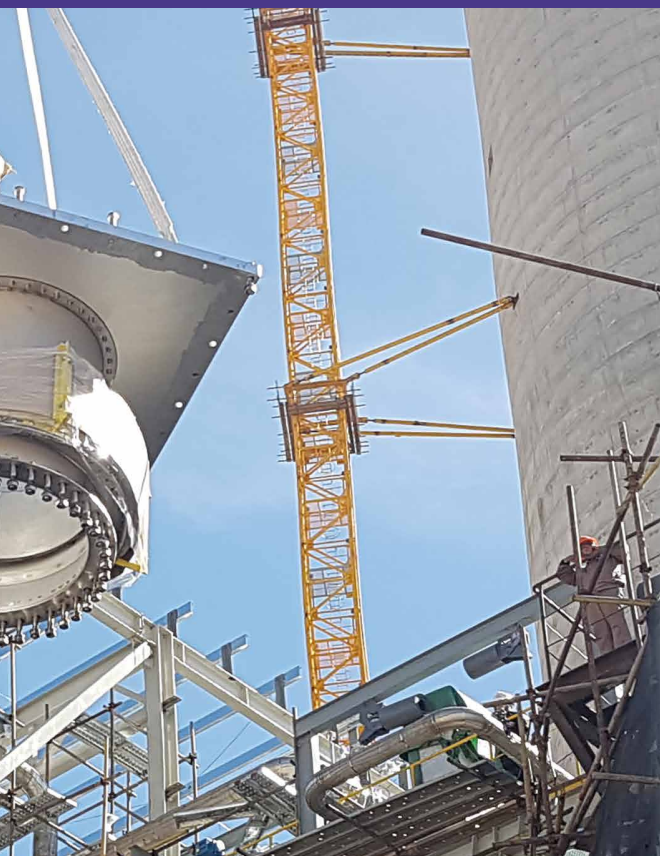
Picture: Installation of the GVSO in a solar power plant
